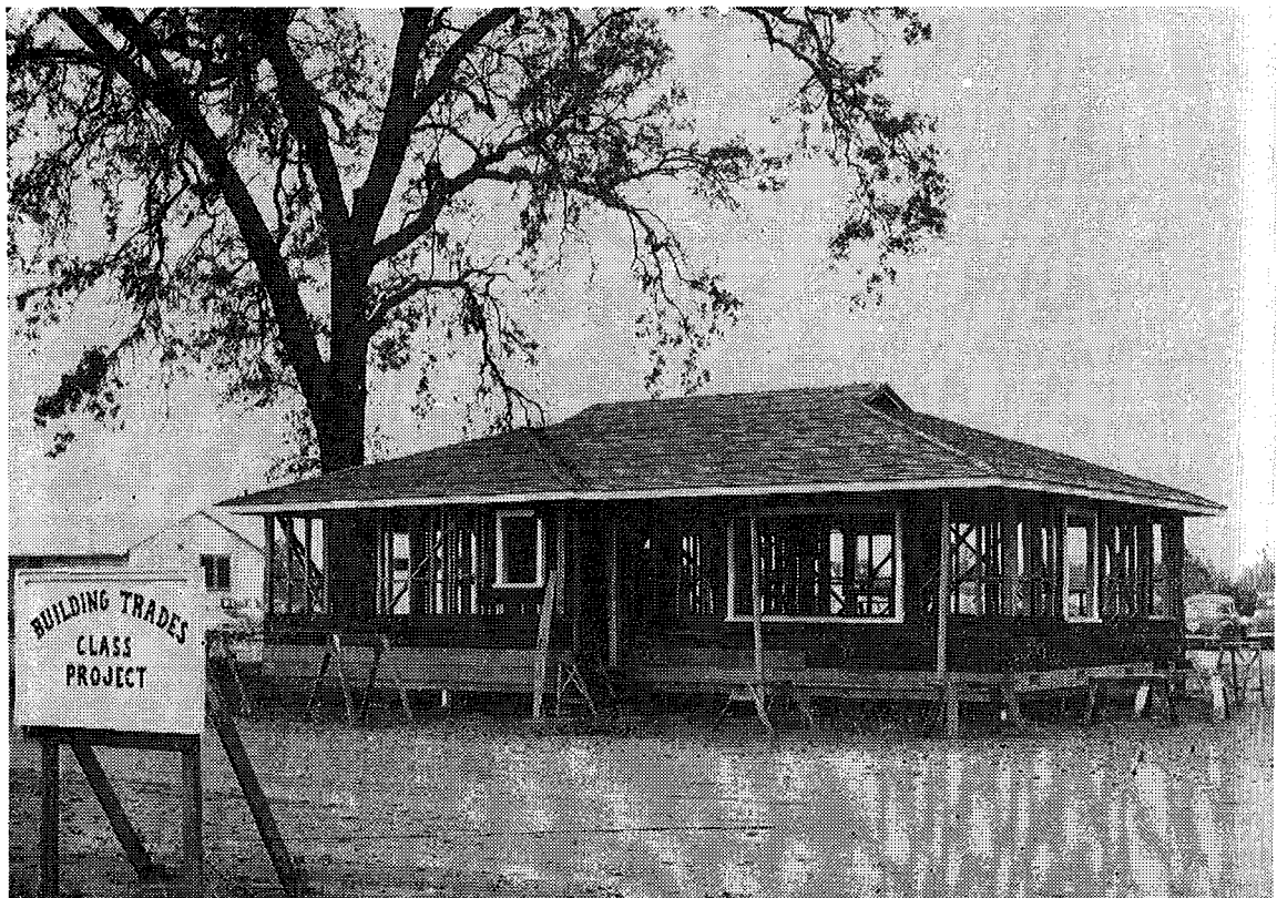
Major construction project of 1950-51 for building trades students
